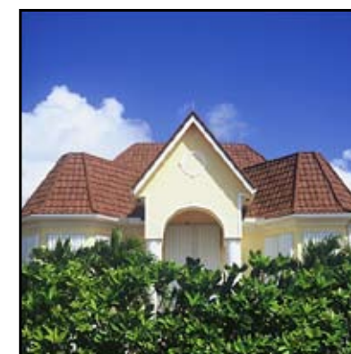
These steel roofs survived hurricanes intact, despite stresses such as falling trees and massive beachfront erosion.
